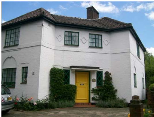
Fig 7.29: No 15 Ickenham Road- at the entrance of Poplars Close
