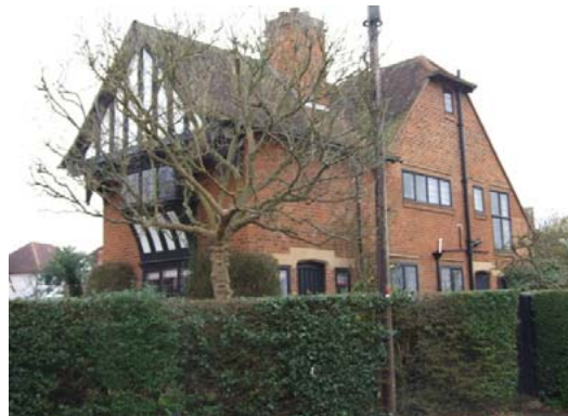
Fig 7.10: The Gables, Church Avenue
