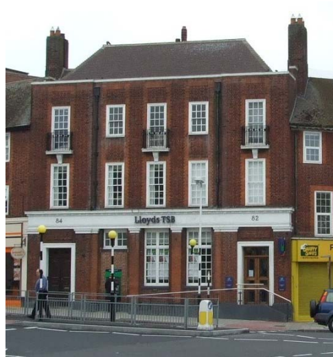
Fig 6.7: Lloyds Bank on the corner with Ickenham Road.
