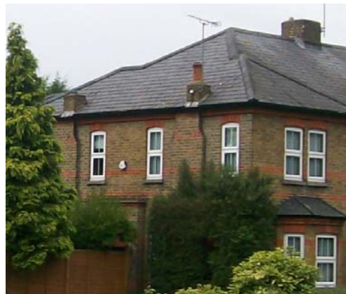
Fig 5.21: Late Victorian semi-detached houses on Bury Street in stock brick with red brick detailing
