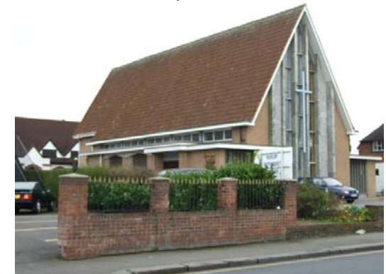
Fig 7.21: Ruislip Methodist Church, Ickenham Road
