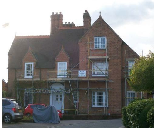
Fig 5.16: Former Vicarage, Deborah Crescent
