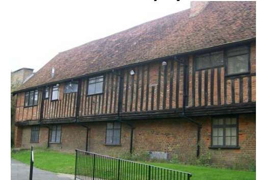
Fig 5.11 Nos 9-15 High Street facing onto St Martin's Church Yard, Grade II*
