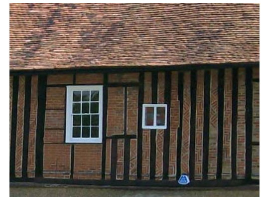
Fig 5.19: Brick noggin - Manor Farm
