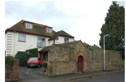
Fig 7.1: Walls fronting No 9 Sharps Lane
