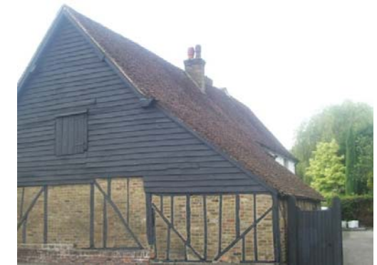
Fig 5.18: Old Mill House- timber framed barn with stained weather boarding
