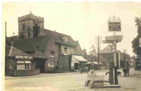
Fig 5.27 Original position of the pump
